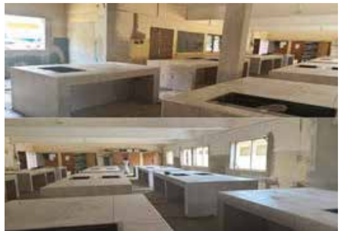
AFTER (work in progress)
